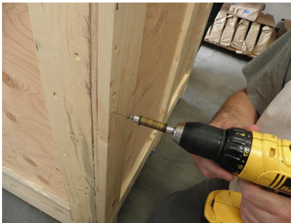
Figure 19. Removing Screws from the Shipping Container
