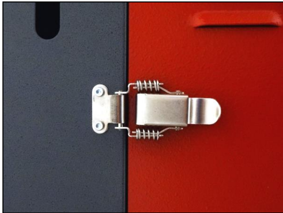
Figure 12. Spring latch for side door
